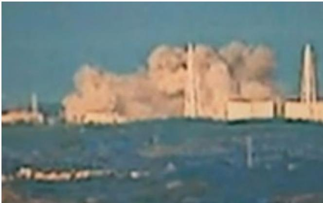
Hydrogen gas leaked out of a reactor, collected under the building's roof and then exploded, blowing the roof off in front of the world's TV cameras. Fukushima had devices called 'recombiners' designed to prevent the hydrogen build-up but they were not working because they needed an external electricity supply.
